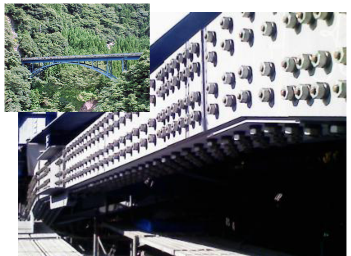
Photograph 11. Strengthening a steel arch bridge
