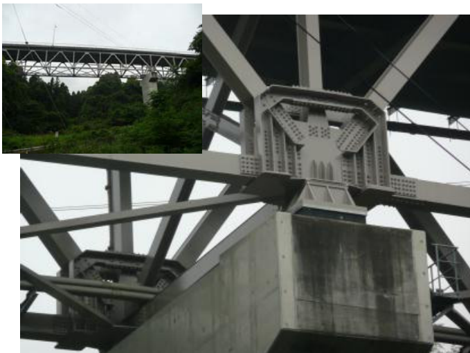
Photograph 14. Strengthening a steel truss bridge
