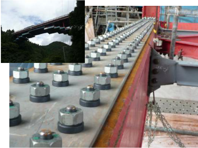
Photograph 12. Strengthening a steel arch bridge
