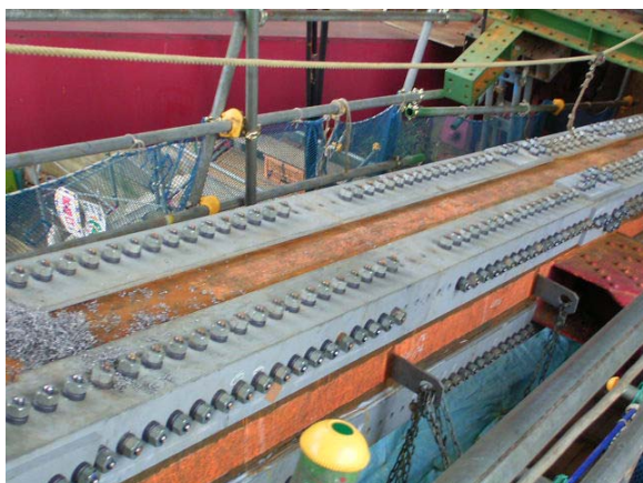
Photograph 2 Strengthening a steel arch bridge
